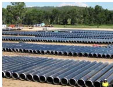
Pipe storage area
