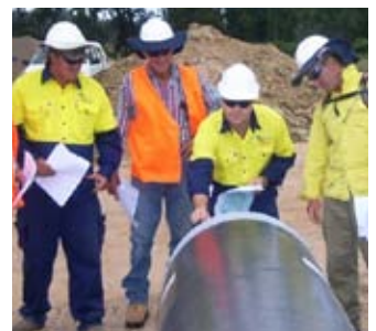
Inspecting the pipe
