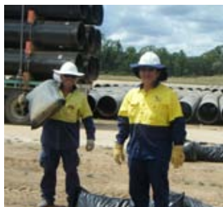
Preparation for pipe delivery
